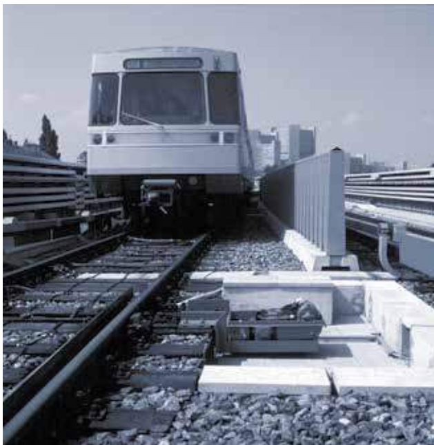
Picture 4: Points Machine along the tracks.
