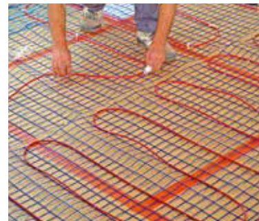
Heating cables connection.
